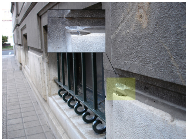
Fig. 3. Location of a black crusted limestone sample in the facade of the historical building.
